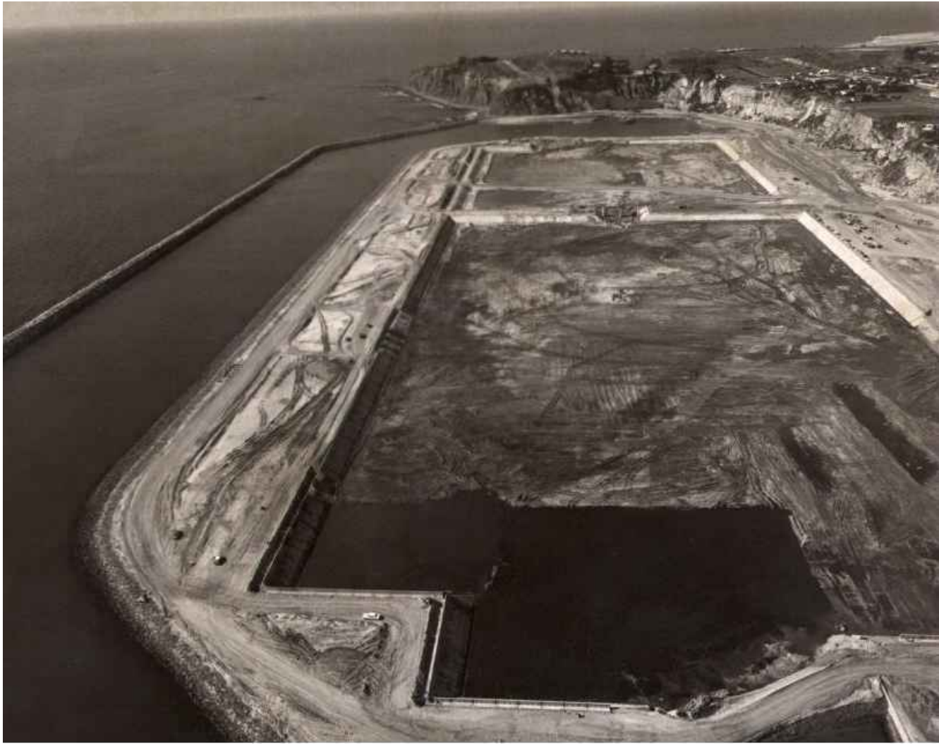
1971 PHOTOGRAPH OF CONSTRUCTION. LIMITED EXCAVATION ACTIVITIES PERFORMED ACROSS MAJORITY OF SITE AS ILLUSTRATED IN CROSS SECTIONS A AND B AND SHOWN IN PHOTOGRAPH.
